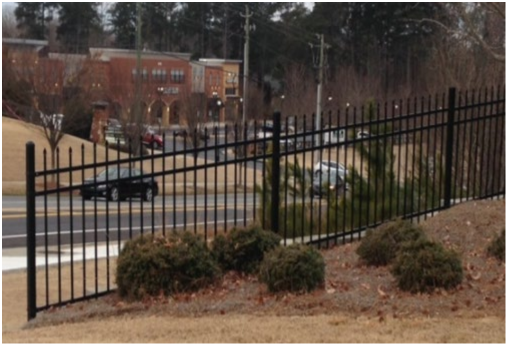
Image 7. For illustrative purposes only demonstrating an example of a raked fence installed on sloping terrain
