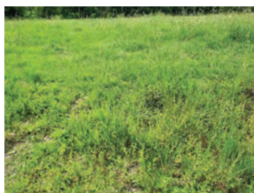
Downstream Right Bank (DRB)
