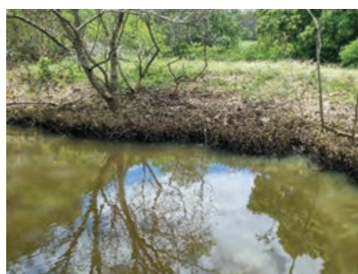
Downstream Right Bank (DRB)
