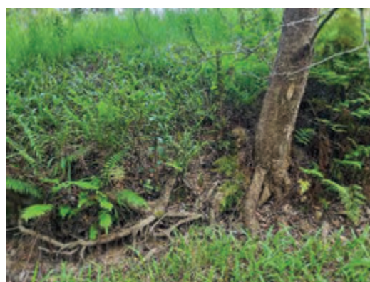
Downstream Right Bank (DRB)
