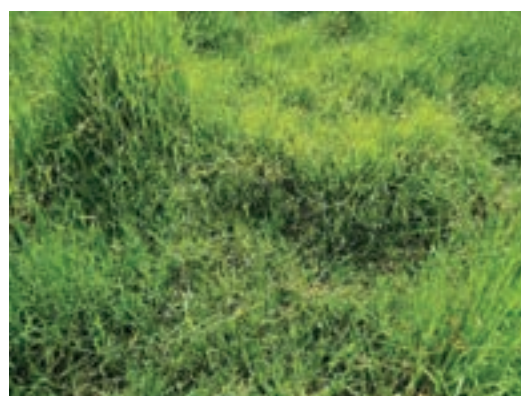
Downstream Right Bank (DRB)
