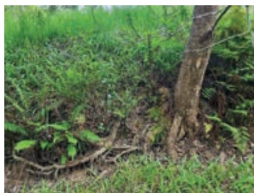
Downstream Right Bank (DRB)
