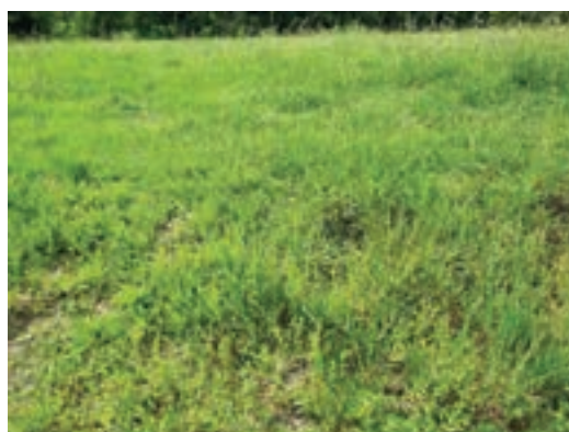
Downstream Right Bank (DRB)
